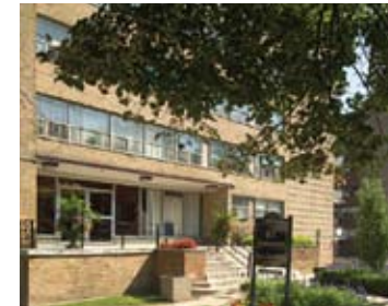
SUITE RENOVATION AWARD UNDER $5000 Metcap Living Management Inc. 87 Jameson
