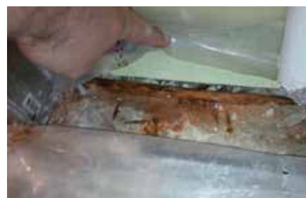
Figure 4 Uncontrolled vapour damage
