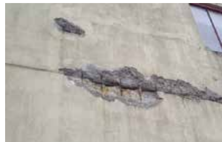
Figure 3 Carbonation, exacerbated by vapour diffusion, concrete spalling
