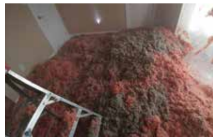
Figure 1 Water damaged ceiling collapse
