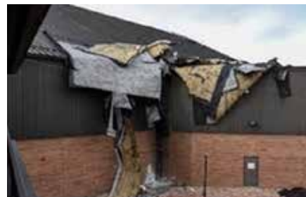
Figure 2 Wind damaged roof
